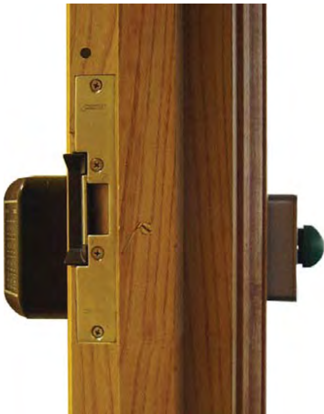
Figure 10.2 Borer Installation At The Door
